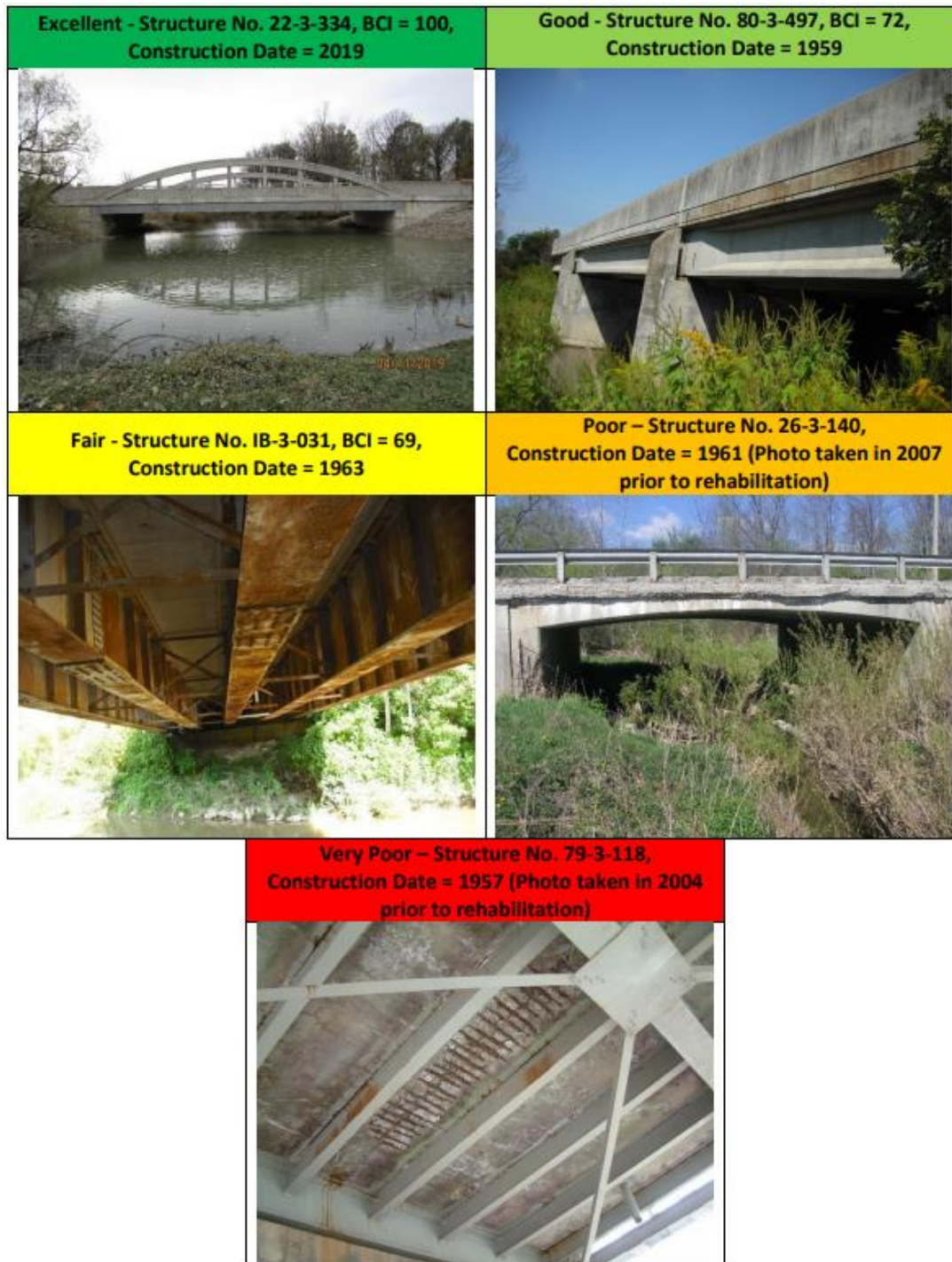
Figure 16: Lambton County – Local Examples of Bridge Condition 24
