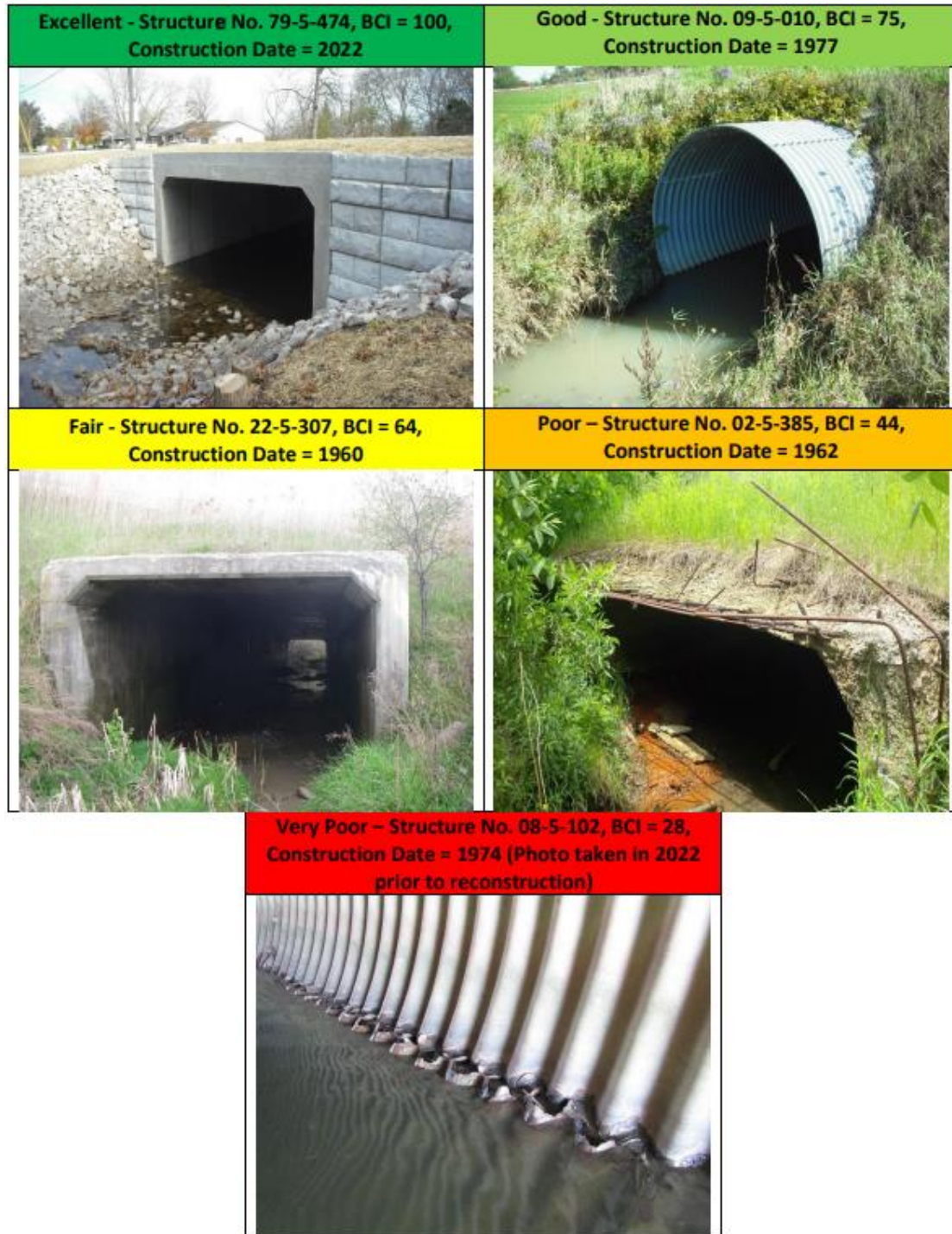
Figure 17: Lambton County – Local Examples of Culvert Condition 25
